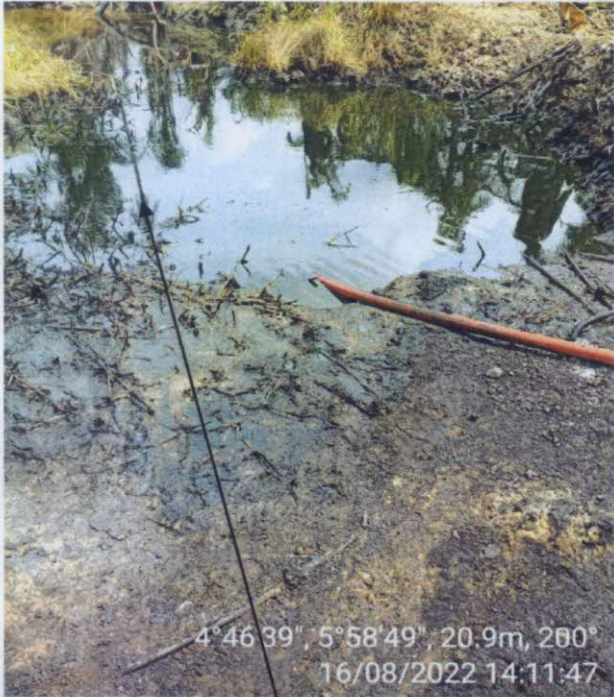
SPILL POINT BEFORE EXCAVATION
